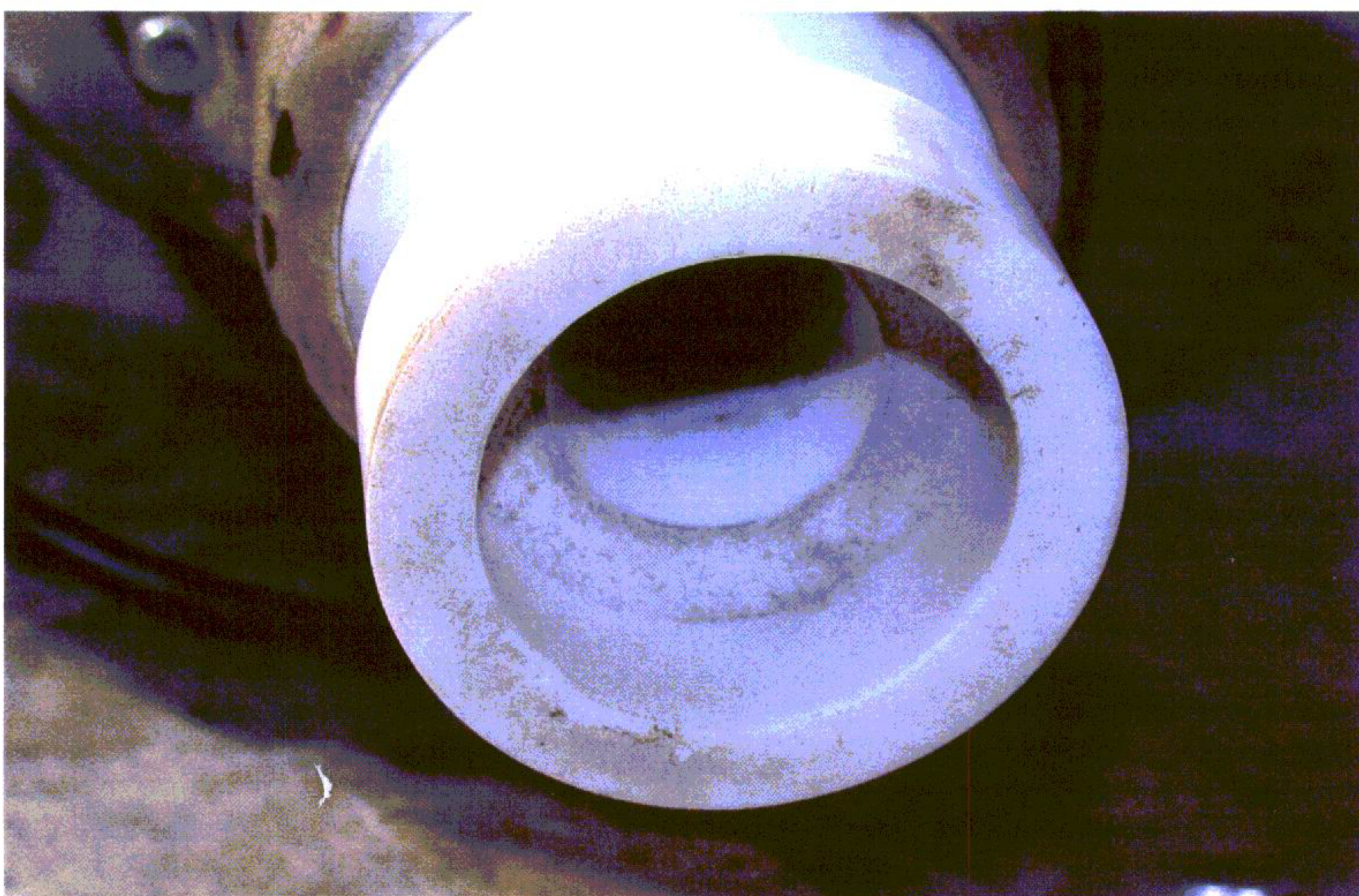
Photo no. 9 Phase S
