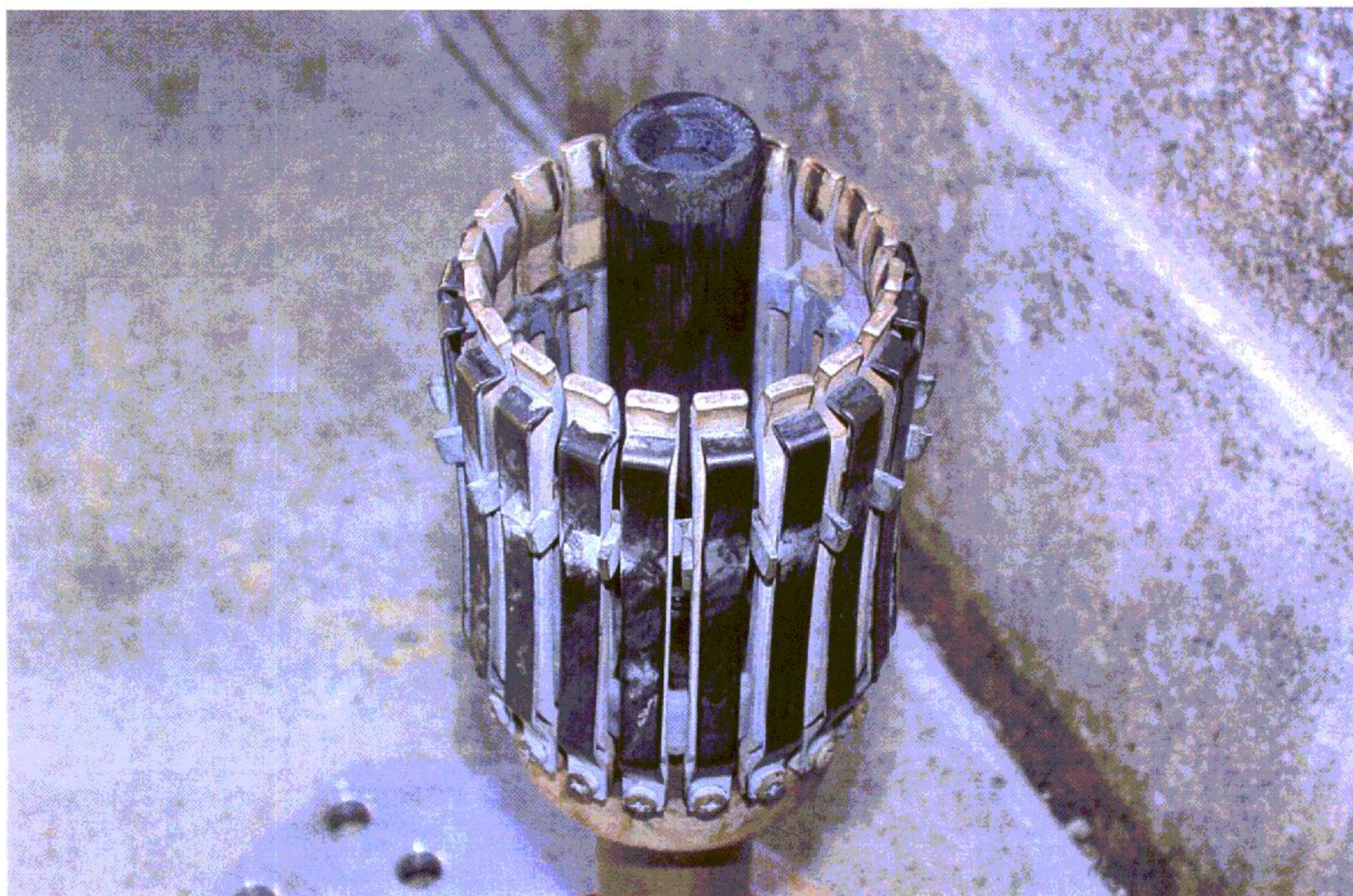
Photo no. 6 Phase S
